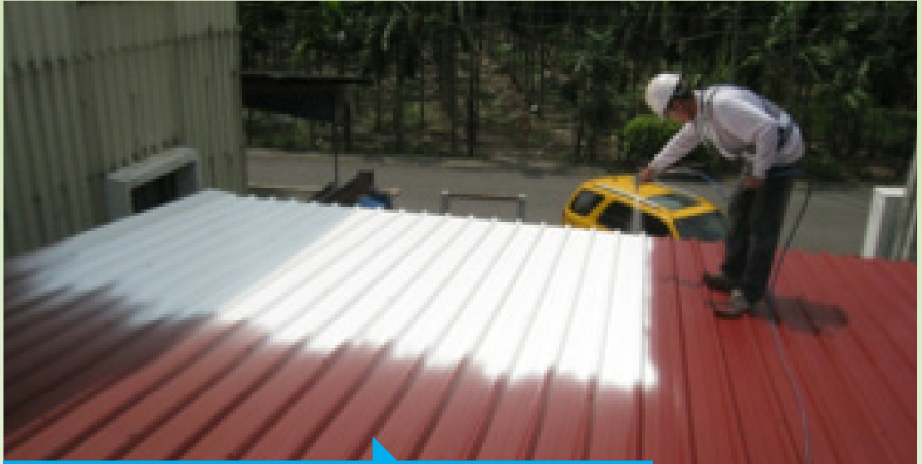
First & Second Topcoat (Adgreencoat, 2 layers, finger touch dry-time around 2hrs)
